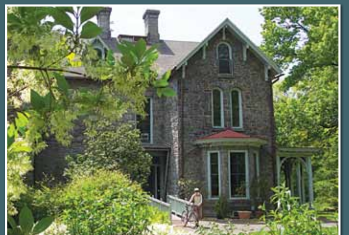
THE FACADE OF THE FRANCIS COPE HOUSE
