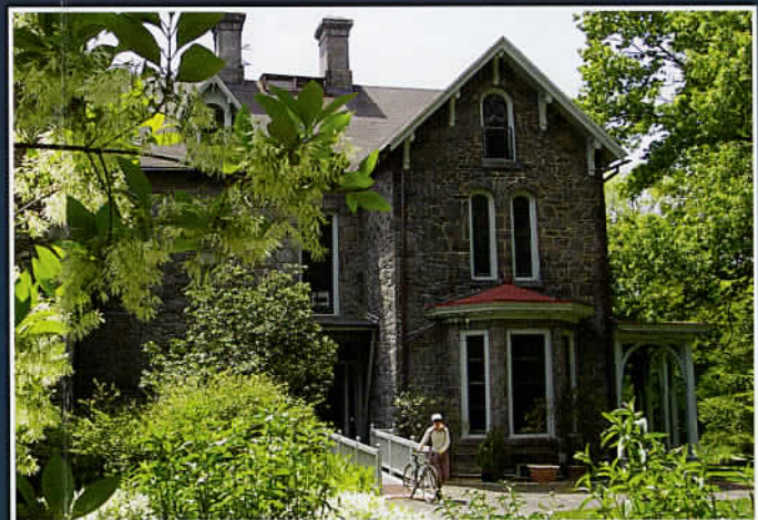
THE FACADE OF THE FRANCIS COPE HOUSE
